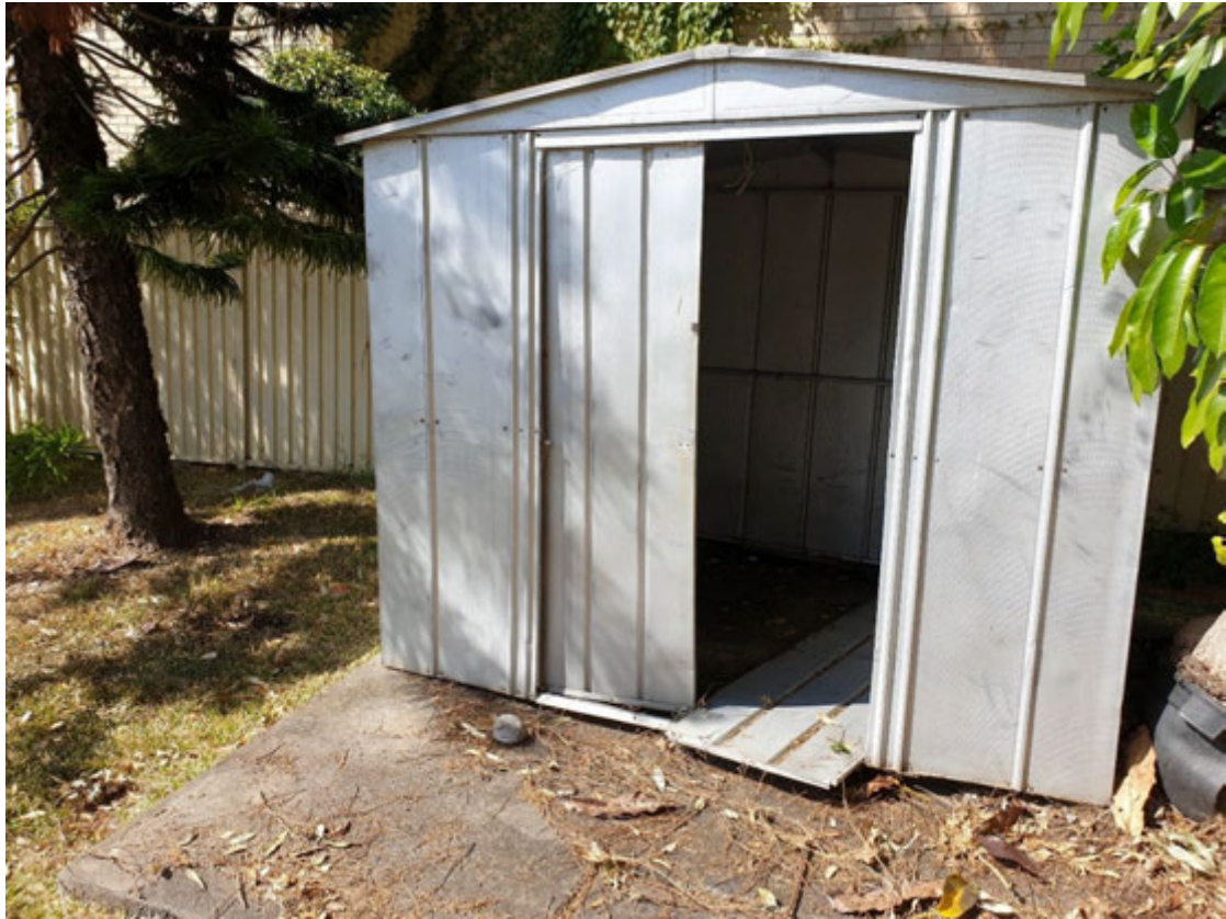
Photograph 5: Zincalume garden shed in rear of 77 Trafalgar Street.
