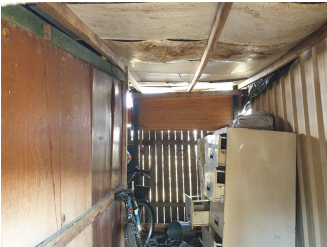
Photograph 10: Compressed timber board construction lean-to attached to metal shed.
